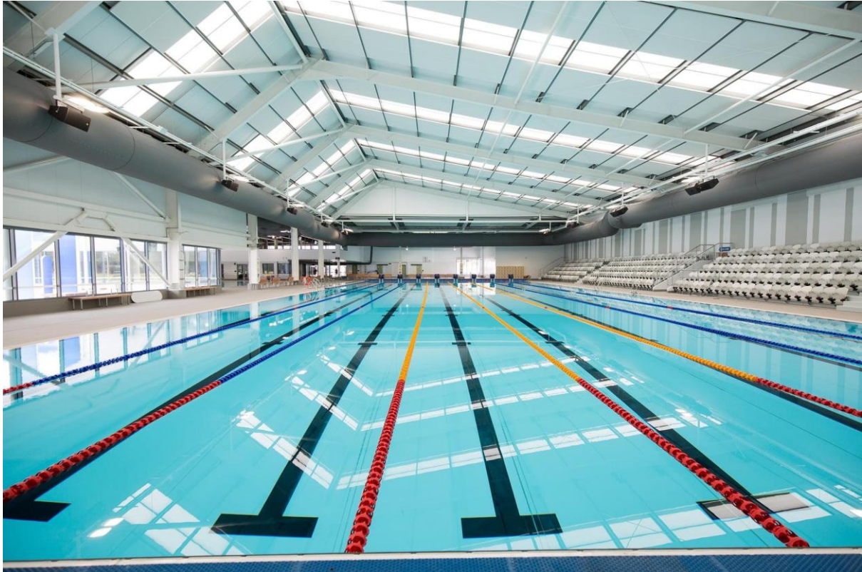
GRAC – 50m pool with a boom. OMEGA touchpads. Additional 25m pool available for warm up/cool down
